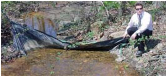
Kneeling by a stream course that drains into Rye Lake from the airport, Parletta inspects a turbidity curtain that helps reduce sediment load in areas that might be disturbed upstream.
